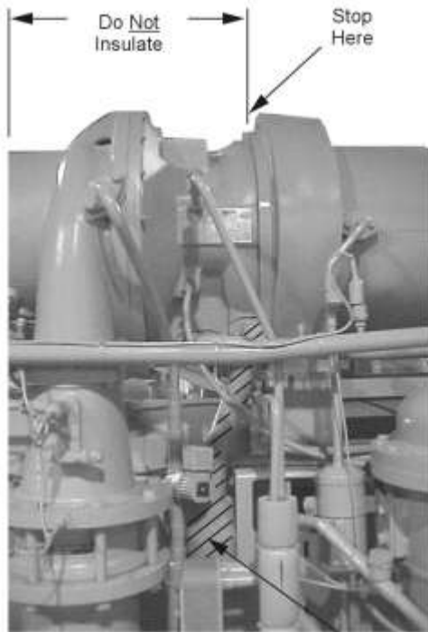
Figure 8, Insulation Requirements, Cooling-only Units
