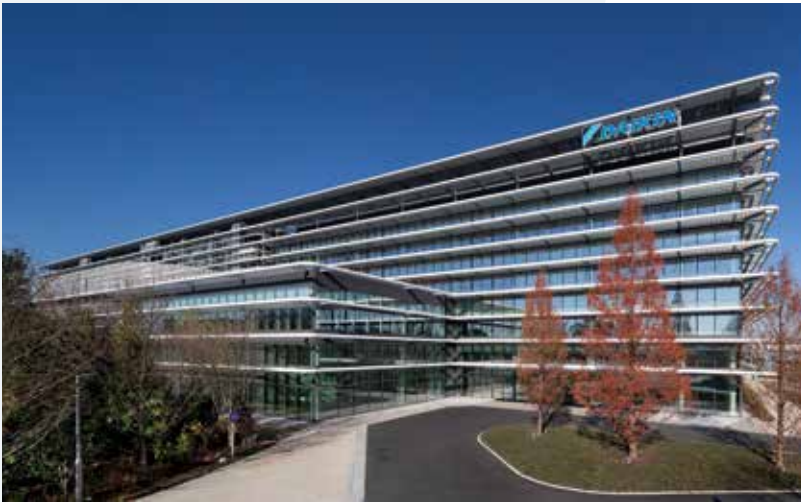
Daikin Technology Innovation Center in Osaka, Japan
