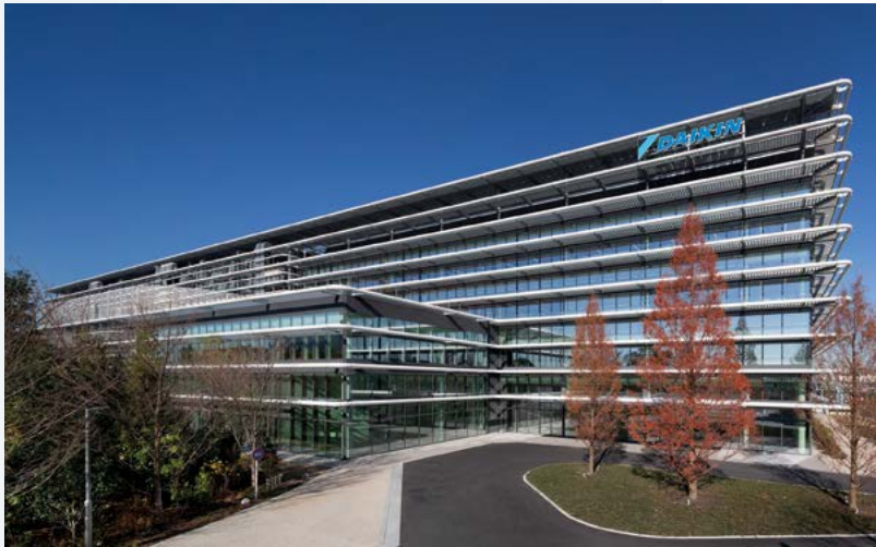
Daikin Technology Innovation Center in Osaka, Japan
